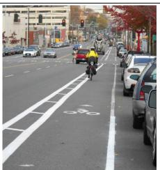
**Buffered Bicycle Lanes** are separate travel lanes designed exclusively for bicycles with painted buffers providing additional separation from the roadway. The buffered space may also include flexible delineators to provide some protection from vehicles. Ideal width: 1.8 m with 0.3 to 0.9 m buffer Minimum width: 1.5 m with 0.3 m buffer (minimum 0.6 m buffer adjacent to parking)
