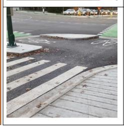
Protected intersections utilize a combination of bicycle signal phases and design elements as well as space allocation to help protect people cycling from turning vehicles. The design of protected intersections include a combination of corner refuge islands, a forward stop bar for bicyclists, a setback bicycle and pedestrian crossing and protected bicycle phasing help protect bicycle users in intersections as they are riding along protected bikeways.
