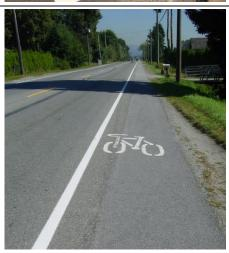
**Shoulder Bikeways** are paved shoulders that are typically found on streets without curb and gutter and where shoulders are wide enough for shared bicycle / pedestrian travel. Shoulder bikeways are typically indicated with the white painted bicycle symbol and with signage alerting motorists to expect bicycle travel along the roadway. Ideal width: 2.0 m to 3.0 m on higher speed roadways. As low as 1.8 m on roadways with speeds of 50 km/h or less. Minimum width: 1.5 m
